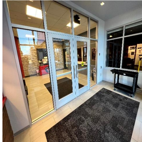
Security Vestibule at Fire Station
