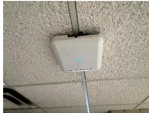
Access Point at Maintenance Facility
