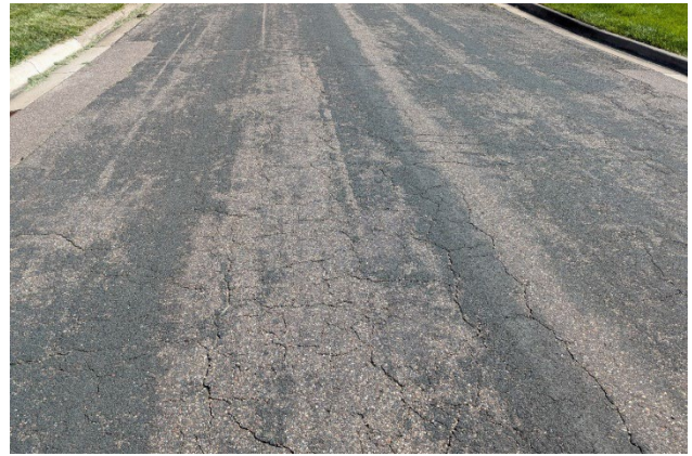
56 PCI (Highclere Drive, north of 130 th Street)
