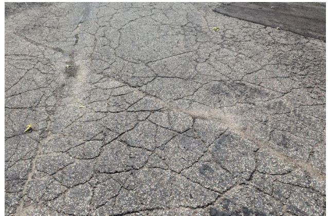
33 PCI (Eagle Ridge Circle, west of Eagle Ridge Drive)
