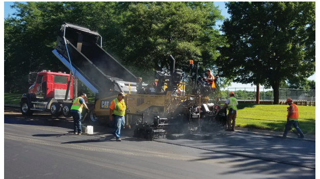
Public Works contractors lay down new asphalt
