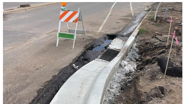
An example of curb repair
