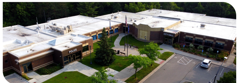
Burnsville Police Department and City Hall
