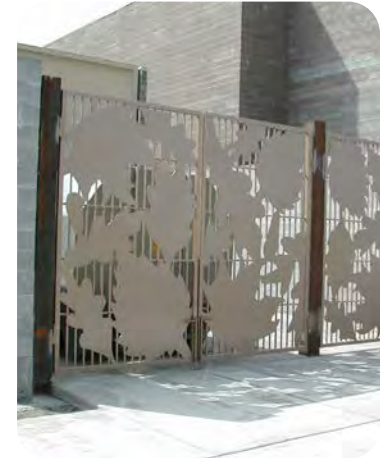
Screening of outdoor trash storage area
