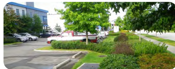
Bioswale continuous along roadway
