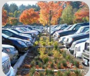
Stormwater management integrated into parking lot
