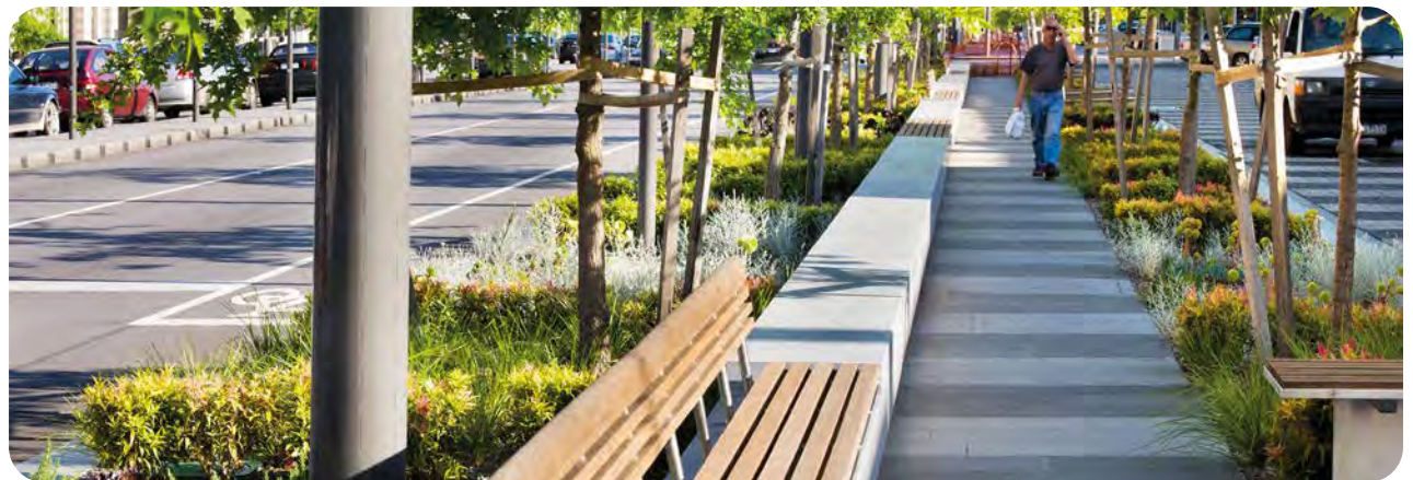
Raingardens integrated into the streetscape public realm (Lonsdale Street, Australia)
