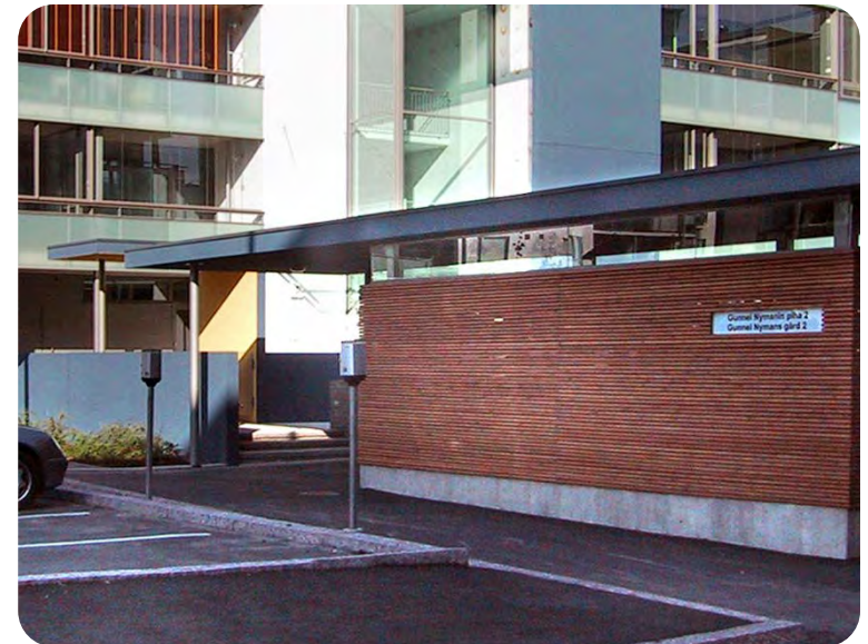
Trash areas should be screened from view and do not negatively impact the appearance of the building or street
