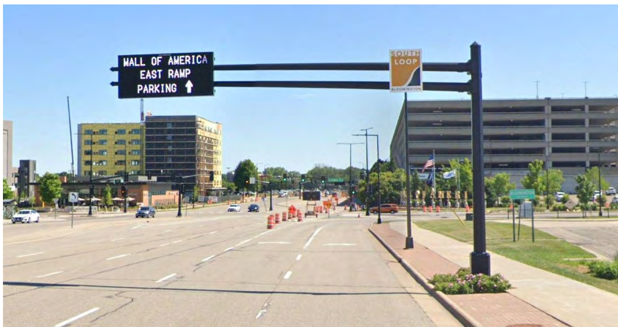
Figure 13 – Dynamic Signage near the Mall of America
