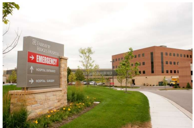
Figure 3-6: Fairview Ridges Hospital
