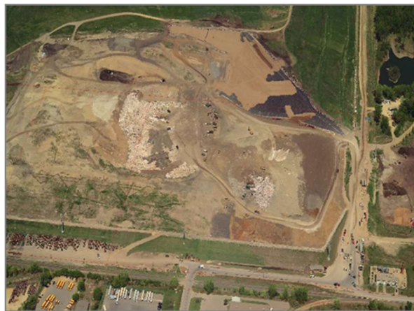
Active Burnsville Sanitary Landfill
